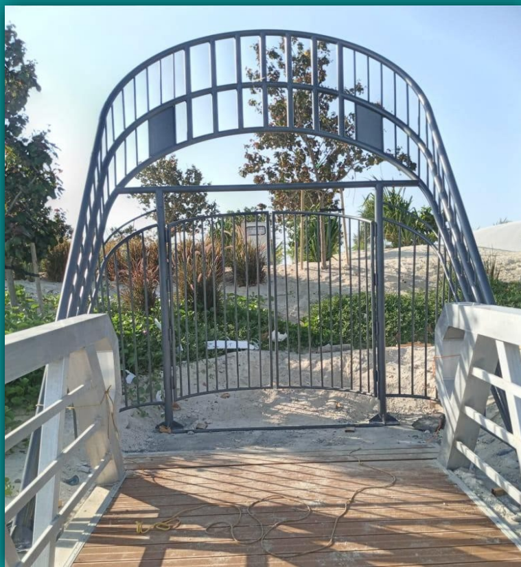
Red Sea – H10 Hatch pier security gate
